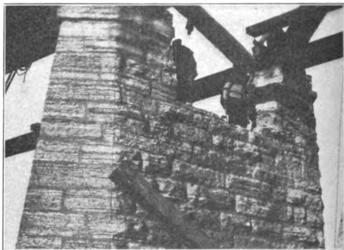
Old Pier Notched to Clear New Girder Span
