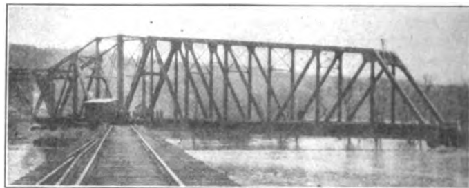
The Draw Span in the Open Position
